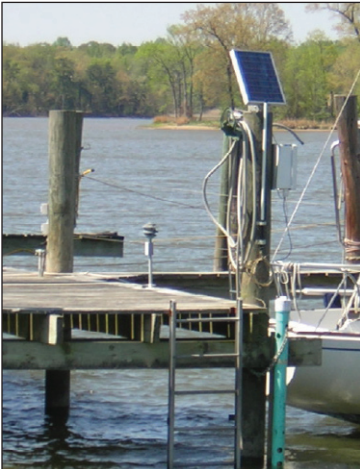
Real-time Continuous Monitoring instrumentation at Lauderick Creek.
