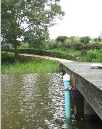
Continuous Monitoring instrumentation is housed in a PVC tube on a pier near Upper Ferry
