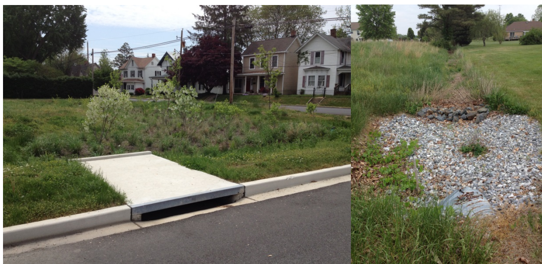
Figure 3-4. Examples of stormwater BMPs in the Corsica River watershed, including a vegetated storm water retention area on the corner of Kidwell and Pennsylvania Ave. (left) and a bioswale system on Quail Run Dr. (right).
